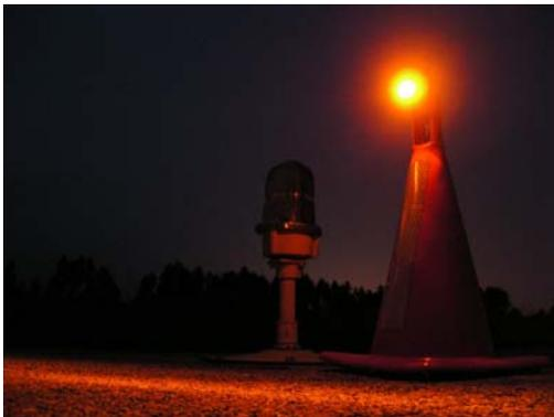
**Figure 2.** A depiction of the low-cost lighting system adjacent to the inactive standard runway lighting.
